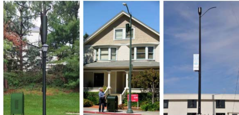
A concept design, left, and two other designs showing how streetlights and utility poles can be modified with equipment, often accompanied by a container on the ground that can be disguised as a mailbox, to deliver 5G cellular signals.
